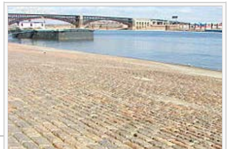
Granite was used for cobblestones on the St. Louis riverfront and for the piers of the Eads Bridge (background). [edit]
